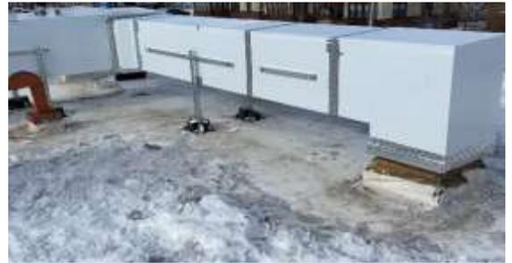
*Installed Q Duct on the roof of the MNATC Stevens Building with Q Rail®, Q Shed®, and Q Lok®.*
