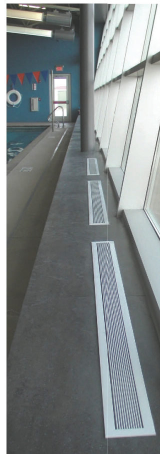
The BlueDuct underground air duct supplies air to the linear diffusers in the natarium area
